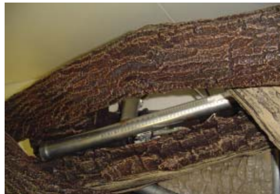
Figure 29A - Installing Back Top Log, Top View
