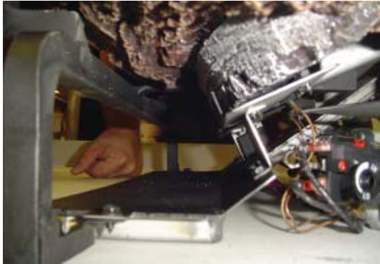
Figure 22C - Installing Right Front Log, Side View
