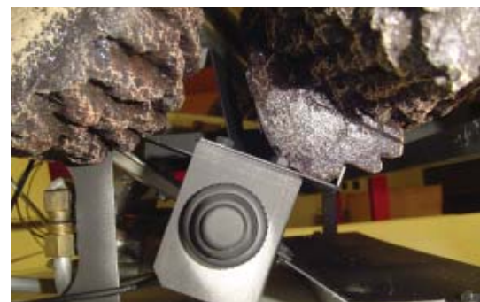
Figure 26A - Installing Front Left Log Side View
