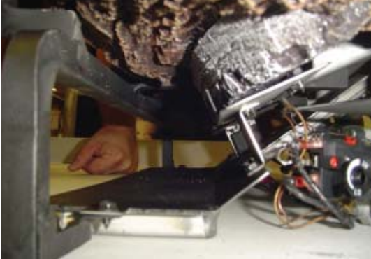
Figure 24C - Installing Right Front Log, Side View
