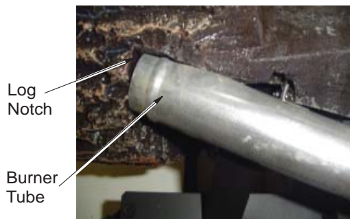
Figure 25A - Installing Back Left Log
