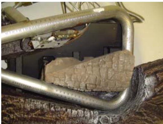
Figure 27A - Installing Charred Log Top View
