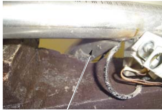
Vertical Portion of Burner Tube
